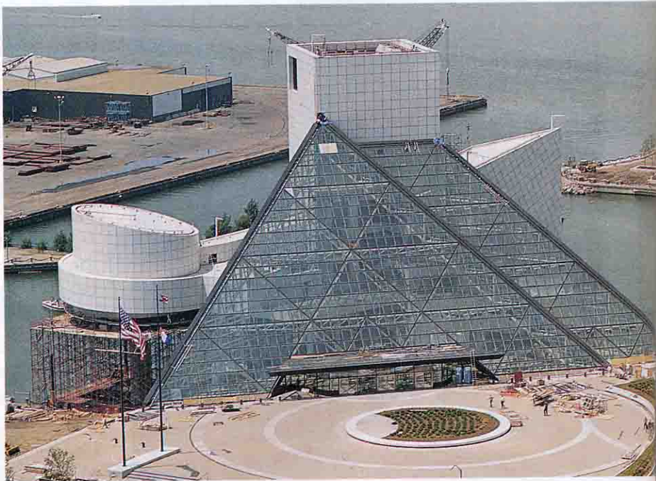
Aerial view of the Rock and Roll Hall of Fame and Museum in Cleveland highlights the sloped-glass "tent" that consists of two sections, one triangular and the other a parallelogram. This sloped curtain wall is supported by 16 bowstring trusses. Photo: Mort Tucker Photography
