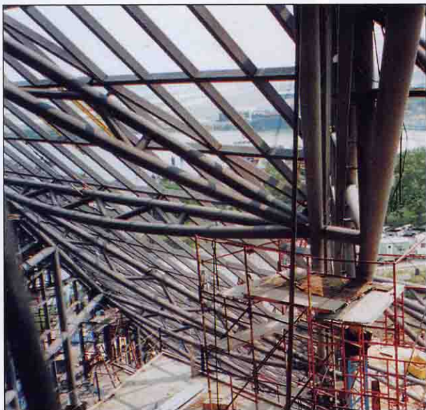
Bowstring trusses are perpendicular to the sloped surface.
