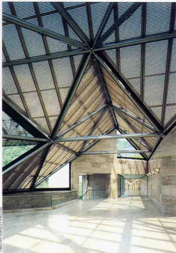
In north corridor (left), horizontal steel members of tetrahedron conceal emergency lighting and uplighting. Typical 19-centimeter-diameter cast-steel node (below) is positioned on center line of module. Wall position is represented by darker line at left.
