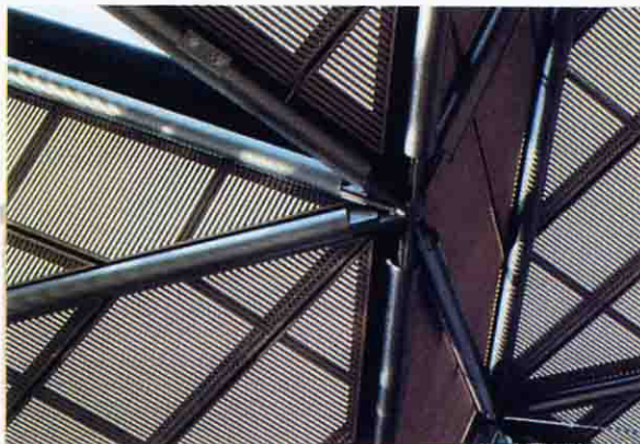
Typical space frame node (above and left) offsets glass and aluminum sunshade layers from structural chords. Peak of space frame (below) rises 1.4 meters above double-height tea court in south wing.
