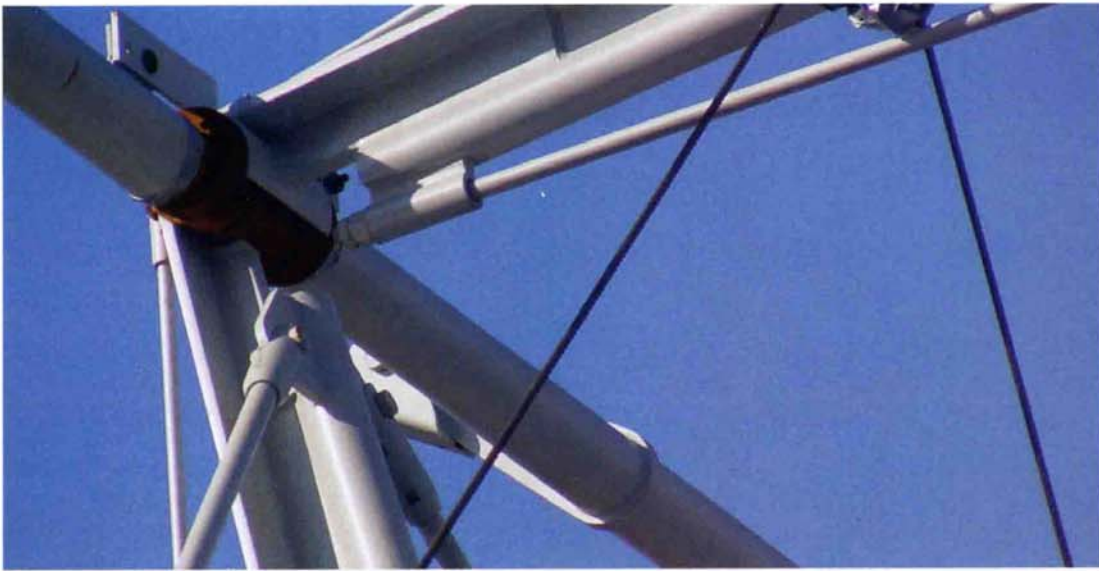
TOP AND MIDDLE LEFT Trusses were site welded to 8-inch pipes running along the top of the columns.
