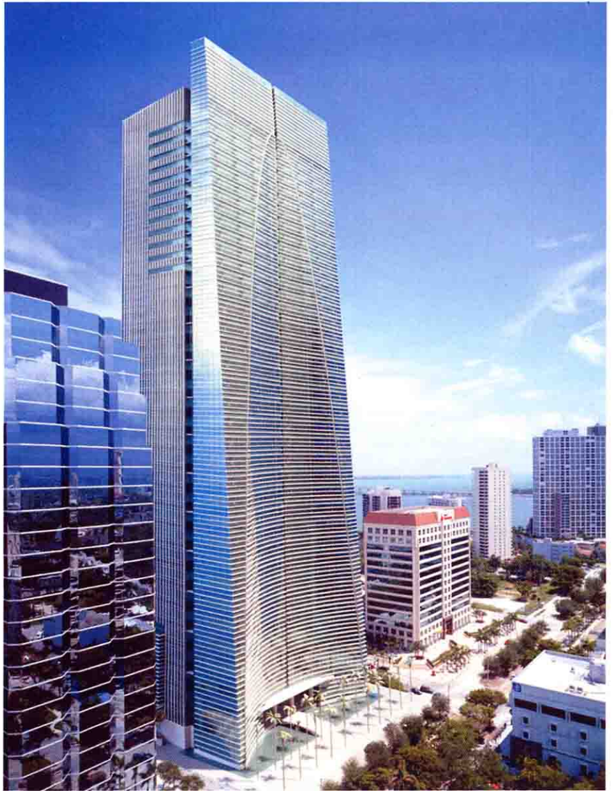
A reinforced curtain wall and ground floor slab are designed to repel floodwaters from the 35-story Espirito Santo Plaza building, under construction near Biscayne Bay in Miami.
