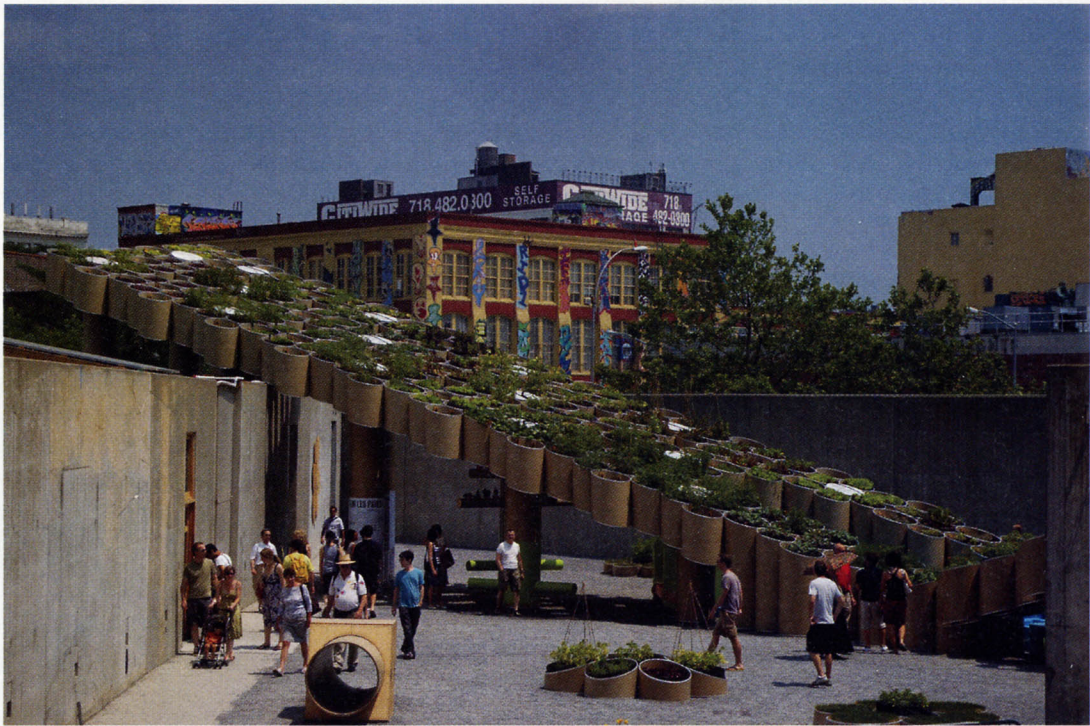
An interconnected cardboard tube structure located in the courtyards of the P.S.1 Contemporary Art Center, in Queens, New York, is supporting a biodegradable “urban farm” that is growing a variety of fruits and vegetables. The temporary structure can be explored by visitors until the end of October.
