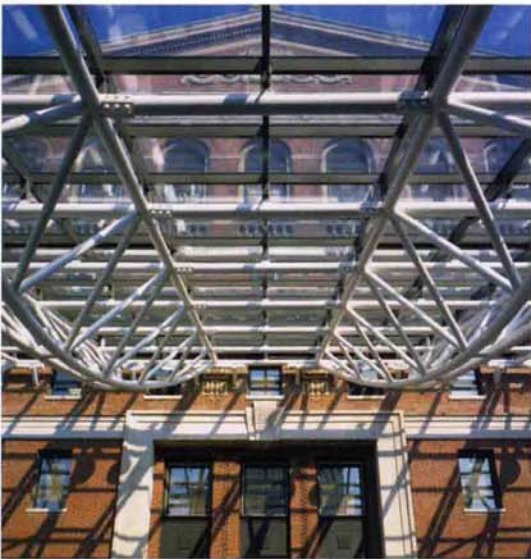
ABOVE The bow trusses, fabricated from 6-inch XXS pipe, support a skylight of Viracon laminated glass.
